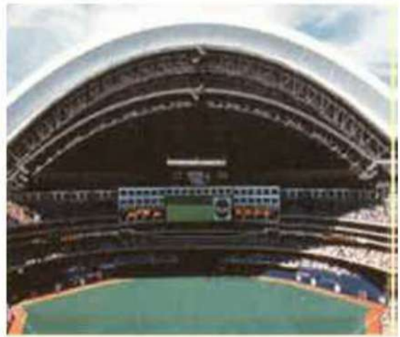
Roof of Skydome in Toronto
